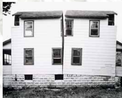
Gordon Matta-Clark, Splitting , 1974, dimensioni variabili, Humphrey Street 322, Englewood, New Jersey
